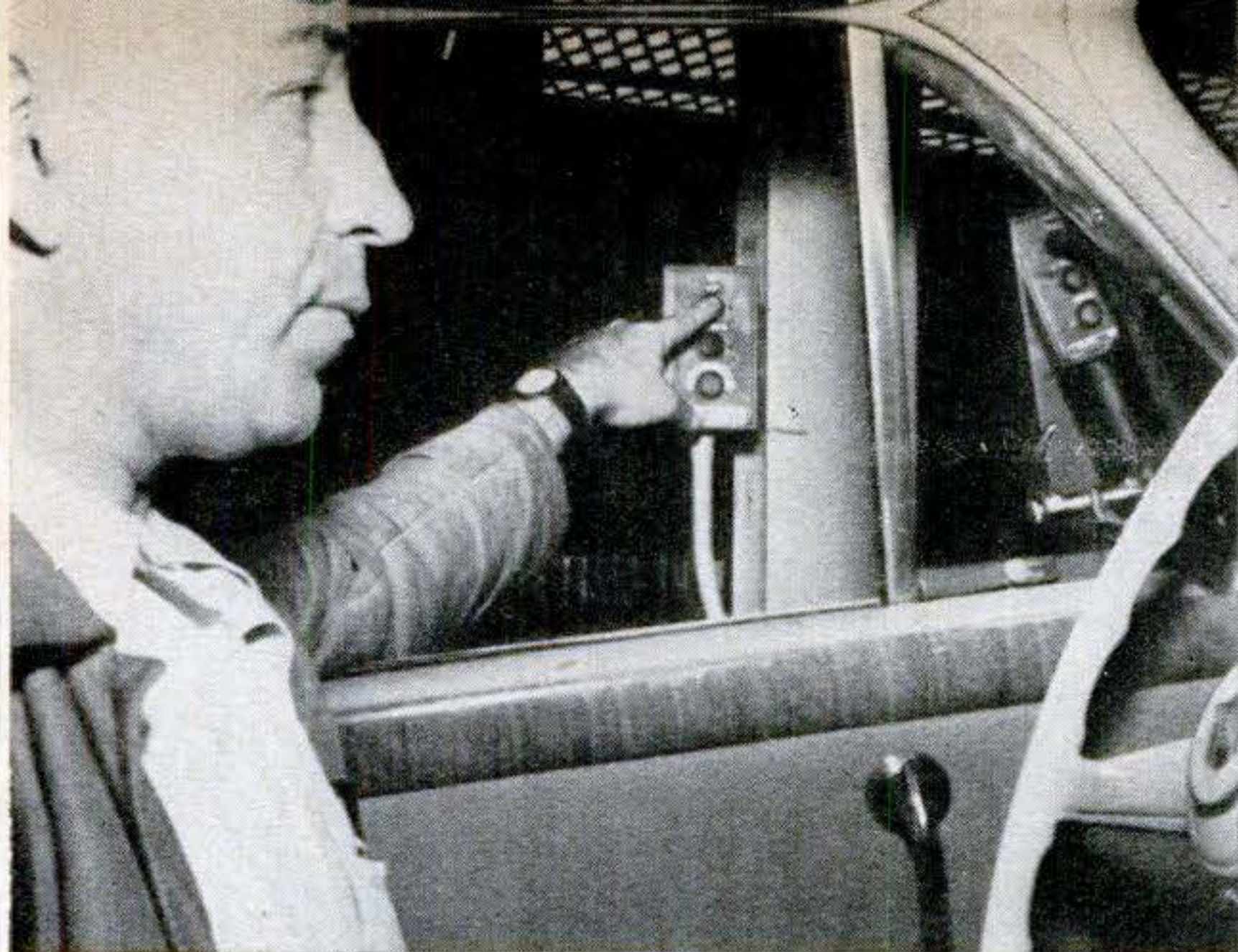
PUSH BUTTONS , operated by attendant from car, lower ramp to connect floors or raise it to let him drive across bridge on same floor.
